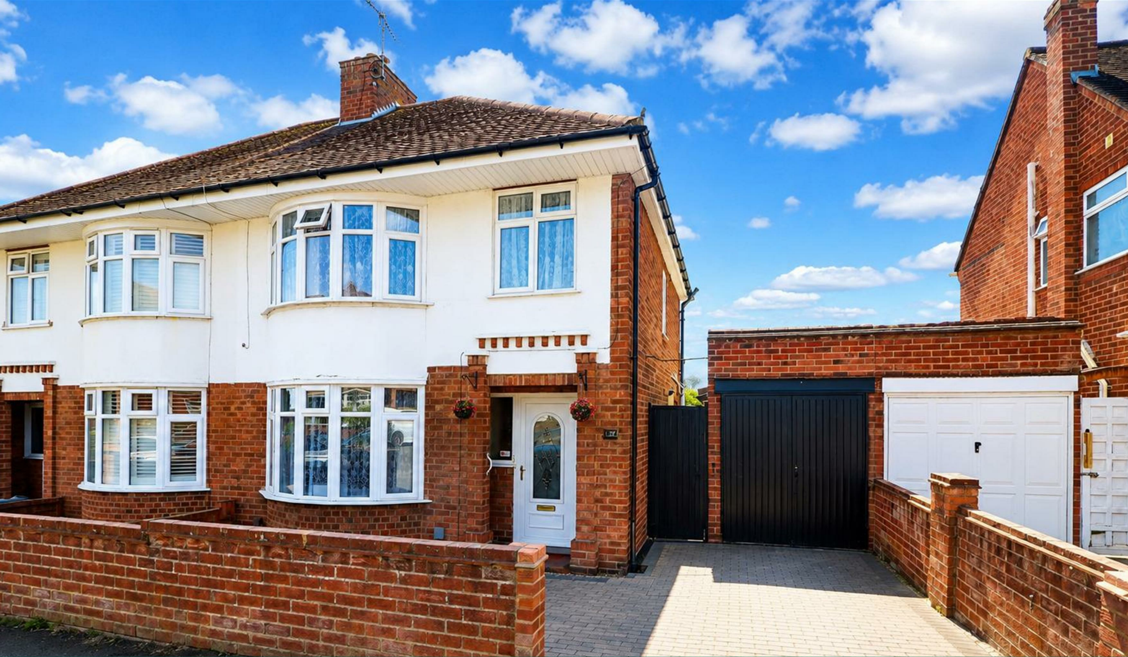
Park Avenue Rushden, Northamptonshire
